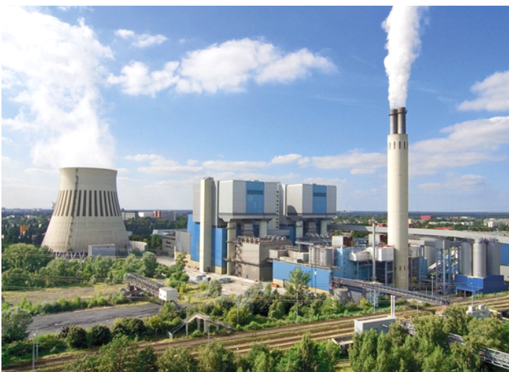
The Reuter West CHP plant in the north-west of Berlin. (Image: Vattenfall)
